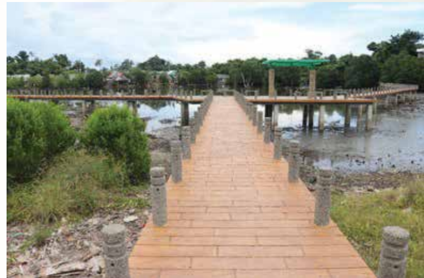
Construction of walkway in Wetland 6
