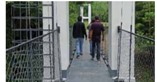
Pimentel Hanging Bridge, Brgy. Pimentel, Diffun, Quirino
