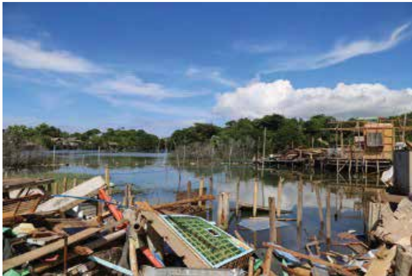
Demolition of illegal structures in Wetland 6
