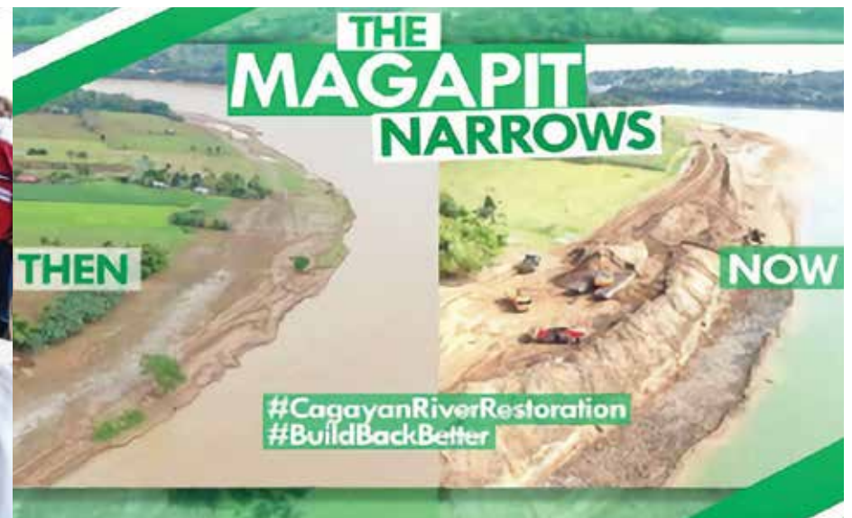
Before and after the conduct of the dredging in Cagayan River
