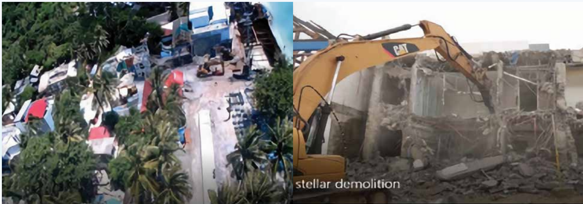
Demolition of Boracay Submarine/Astoria Stellar Hotel in 2018 (L to R)
