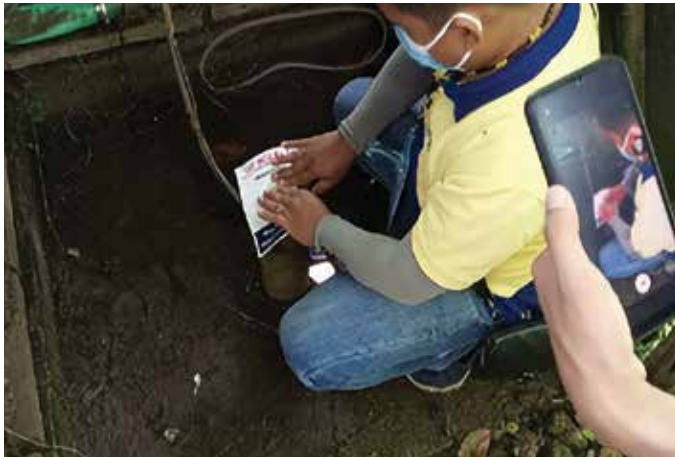
Temporary sealing of well located at 13-A, Navy Base Road, St. Joseph Village, Baguio City
