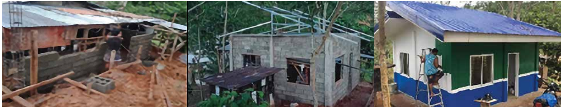
Renovation of PTFNR Satellite Office located in Mabatas, Upper Ulip, Monkayo
