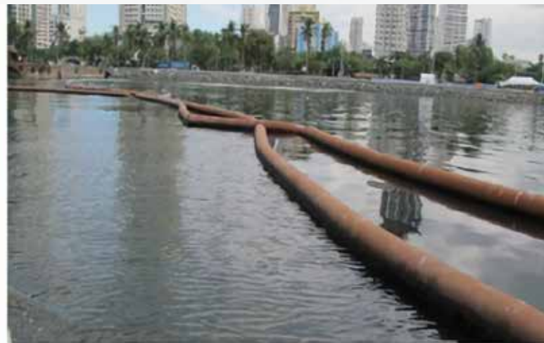
3,100 linear meters of silt curtains
