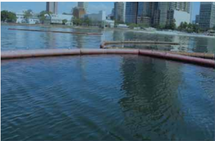
3,100 linear meters of silt curtains
