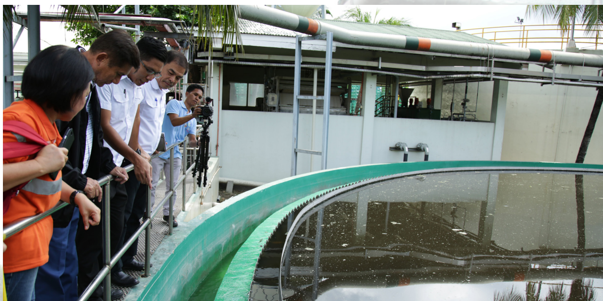
Sec. Cimatu, with EMB-NCR Regional Director Vizmindia Osorio (extreme left) inspects San Miguel Brewery-Wastewater Treatment Facility in Valenzuela City.
