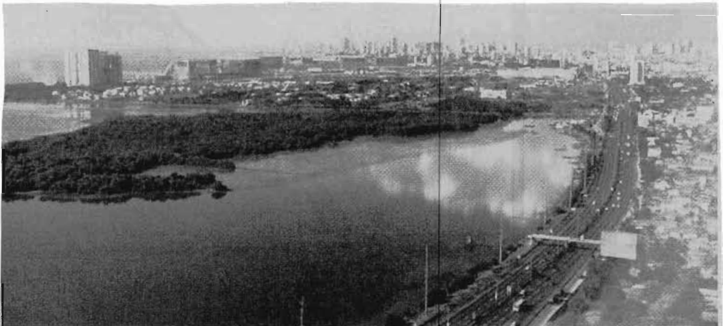
A VIEW of the Pasay City coast of Manila Bay and the Cavite coastal road tollway. The Pasay local government unit has allotted rights to reclaim the waters under its jurisdiction, while the consortium will shoulder the costs including raw land reclamation works and expenses.
