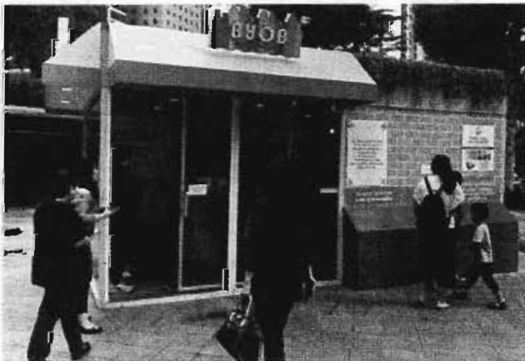
The BYOB store is made of eco-bricks that use plastic discards as a component.
