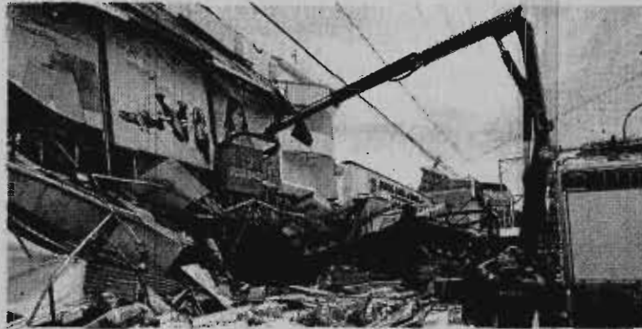
DAMAGE The 6.5-magnitude earthquake that hit Davao del Sur province last year destroyed homes and buildings in Digos City. —BONG SARMIENTO
