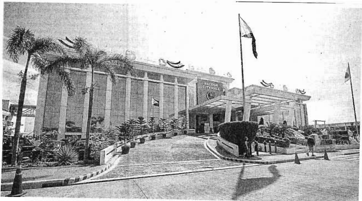
NEW City Hall of Bacoor attests to the progress of the city achieved through good governance and adherence to the principles of sustainable development.
