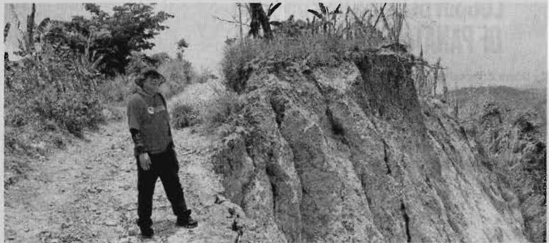
DANGER ZONE The Mines and Geosciences Bureau (MGB) says the mountain village of Diaz in Porac town, Pampanga province, is susceptible to landslides, as shown by eroded roads leading to the Aeta community. —PHOTO COURTESY OF MGB CENTRAL LUZON
