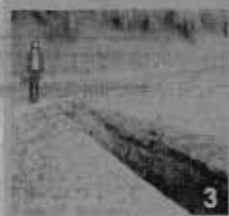
A fissure with a vertical displacement of 30 to 40 cm cut the road parallel to the seashore in Brgy. Bilbinwang, Agoncillo.
