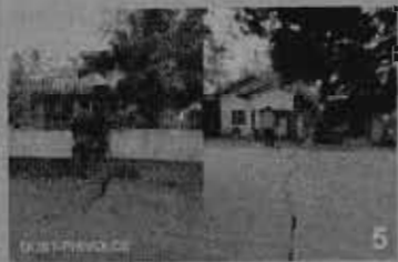
Along the Lemery-Agoncillo Road in Brgy. Dayupan, Lemery, northeast-trending fissures were measured with a vertical displacement of 29 cm. Widening of fissures by ~5cm was also documented.
