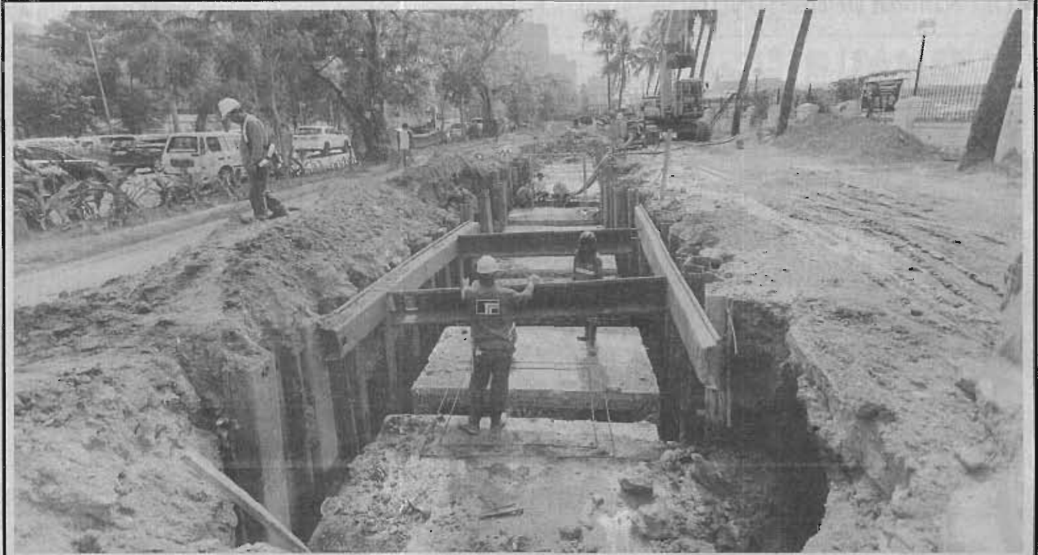
WASTE-FREE MANILA BAY Construction workers along Roxas Boulevard work over the weekend to finish a drainage system to prevent waste from polluting Manila Bay. PHOTO BY ENRIQUE AGCAOILI
