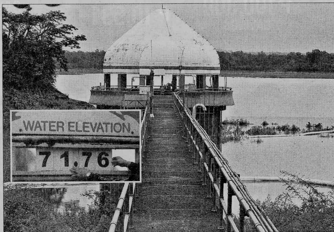
After rains brought by Tropical Depression Egay, water elevation in La Mesa Dam continues to rise (inset).
