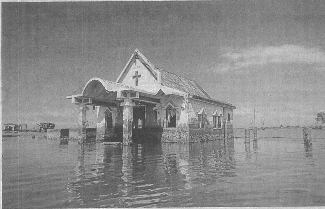
SCENE OF SUBSIDENCE Groundwater pumped out from unregulated wells has caused subsidence, resulting in sinking areas, like this village in Pariahan, Bulakan, Bulacan province. —AFP
