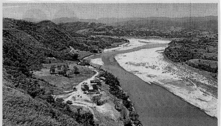
CHANNELING WATER The site of the Chico River Pump Irrigation Project in Kalinga province. Proponents say more than 7,500 hectares of rice farms in Cagayan province and 1,170 ha in Kalinga stand to benefit from the Chinese-funded irrigation system. —PHOTO COURTESY OF CORDILLERA PEOPLES ALLIANCE
