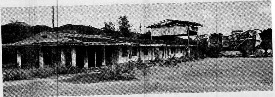
Abandoned Building. A run-down office Building inside the Marcopper mining area, abandoned in 1997, after Placer Dome, Inc. left the Philippines following the mine spill.
