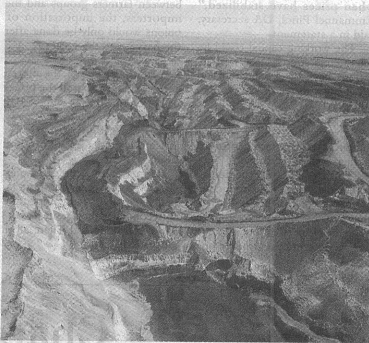
Backfilling ongoing. From an elevation of -260 meters - the equivalent of a 78-story building - the southern portion of the pit is now flat.
