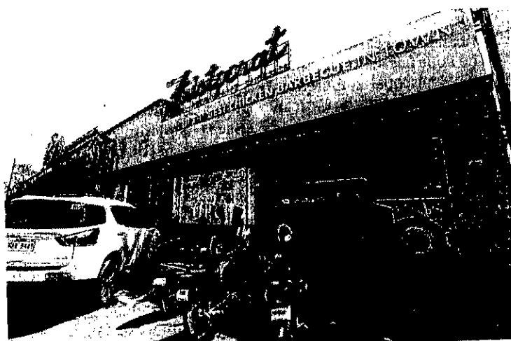
NOTICE OF VIOLATION Aristocrat Restaurant along Roxas Boulevard is among the restaurants issued cease-and-desist orders by environment authorities for polluting the bay.
