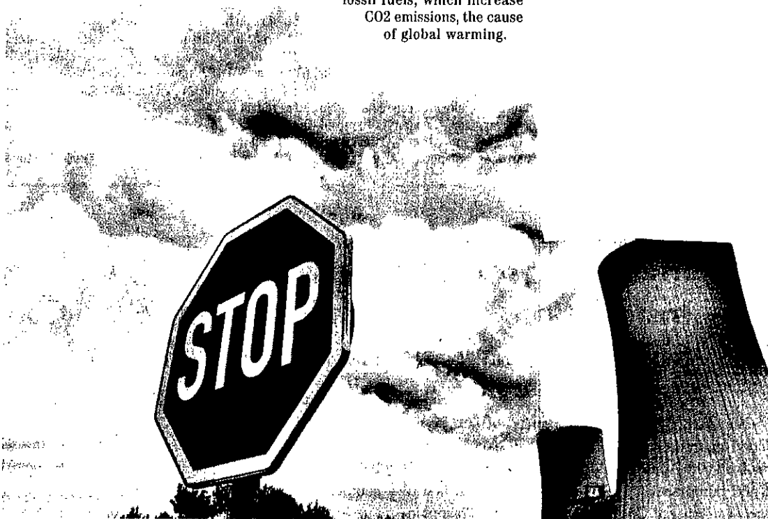
The power plant "Neurath" run by coal from the brown coal open cast mine Garzweiler is pictured in Rommerskirchen, west Germany. Smoke from factories is one of the major causes of air pollution.
