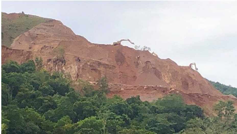
(Quarrying operation in Mt. Dipulao, Barangay 6 Coron. Contributed photo)
