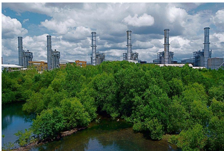
A First Gen Corp natural gas plant is shown in this photo from the company's website. Handout photo
