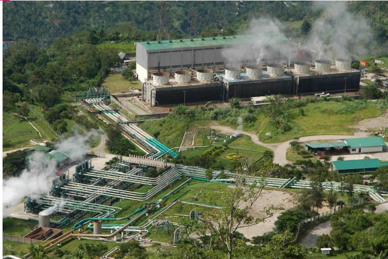
Palinpinon geothermal plant in Leyte (Photo: First Holdings)
