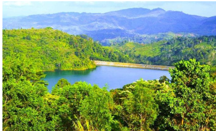
The Sulphide Dam at the Canatuan mine.
