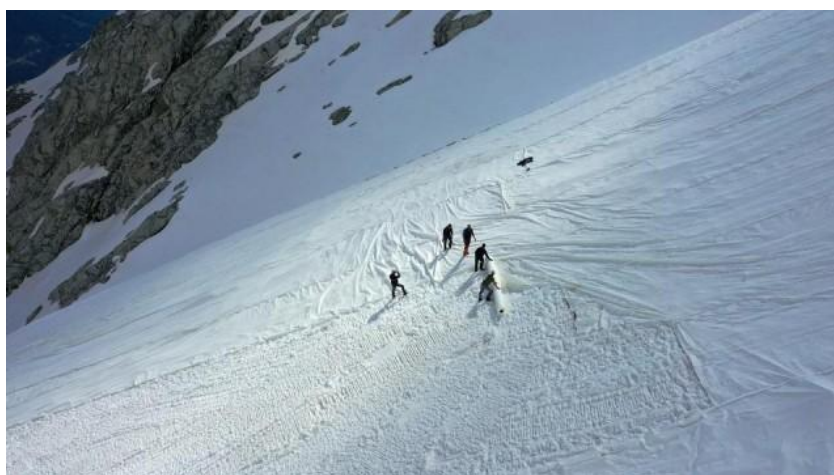
An aerial photo taken on June 19, 2020 shows workers covering with huge geotextile sheets the Presena glacier (2700m-3000m) on the Val di Sole near Pellizzano in Trentino, northern Italy, in order to delay snow melting on skiing slopes. Miguel Medina/AFP
