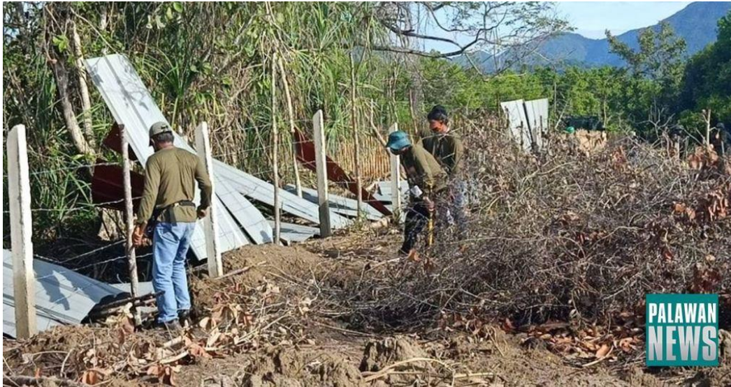
(Demolition on the mangrove area allegedly owned by P/Col. Marion Balonglong.)
