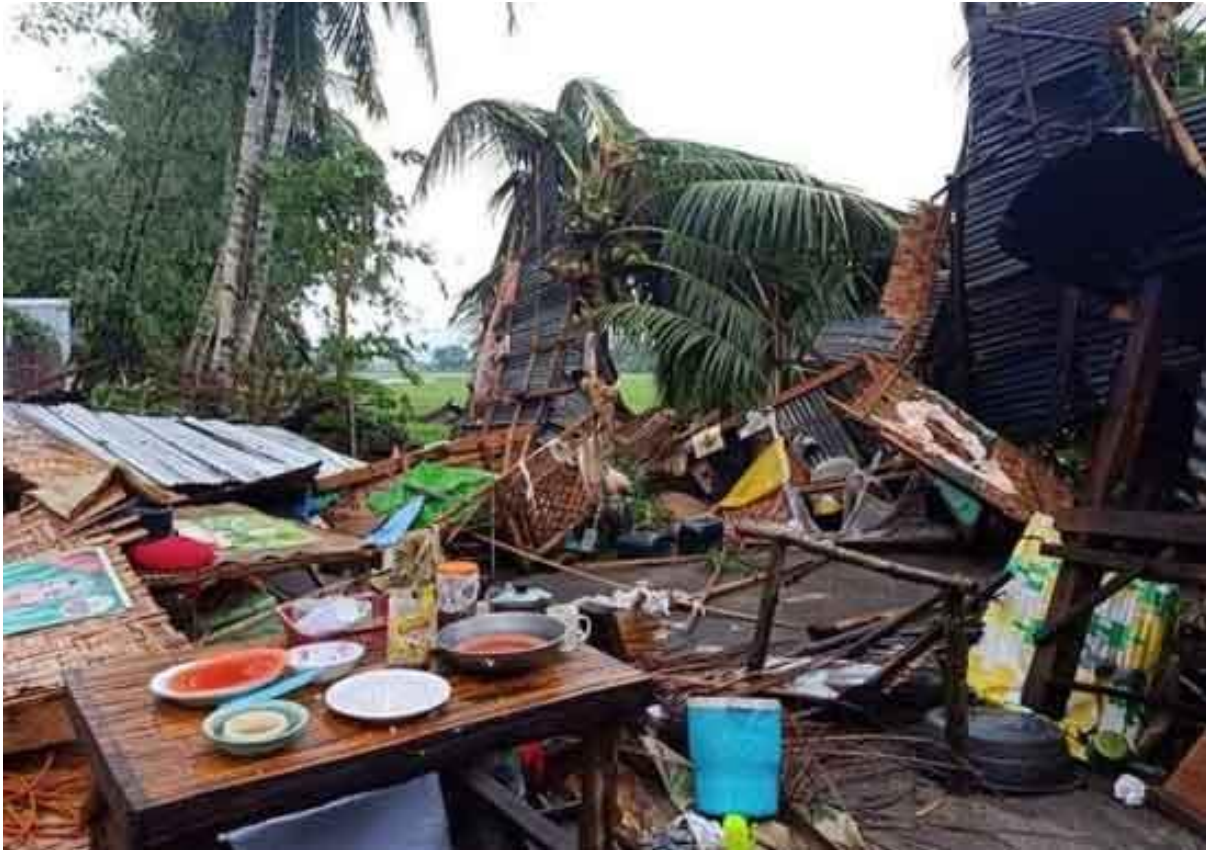
At least 40 houses, made from light materials, were damaged by a tornado that hit farming communities in President Quirino, Sultan Kudarat over the weekend of June 7, 2020 as torrential rains hit the province. Affected villages were Romualdez and Kalanawi 2. The local government has already extended help to the victims. PHOTO BY ASANGAN T. MADALE/CONTRIBUTED PHOTO
