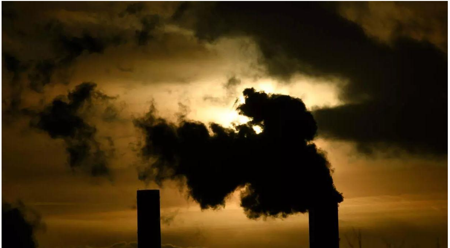
A coal power plant of German energy giant RWE in Weisweiler, western Germany, on January 29, 2020. © Ina Fassbender, AFP
