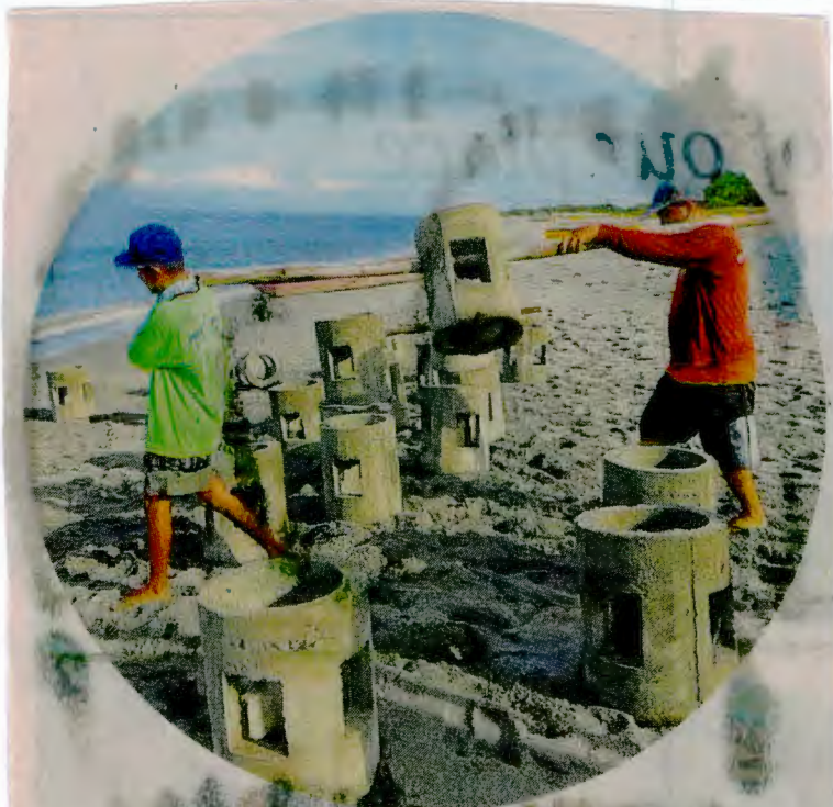
These concrete barriers make up the artificial reef that was installed in Barangay Panan in Botolan, Zambales.
