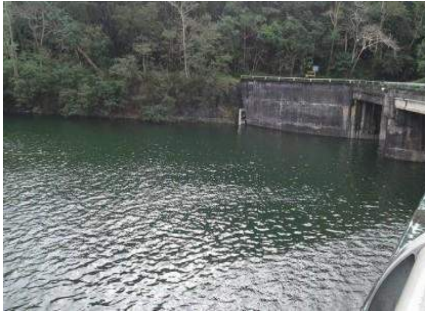
Angat dam (File photo)
