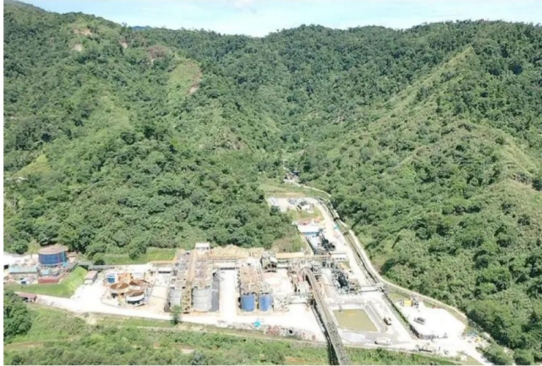
The facilities of the FCF Minerals Corp. in Runruno, Quezon, Nueva Vizcaya. CONTRIBUTED PHOTO
