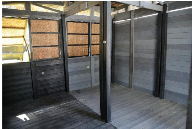
A view of the shelter made out of eco-lumber at The Plastic Flamingo upcycling facility in Muntinlupa City on March 18, 2022. George Calvelo, ABS-CBN News
