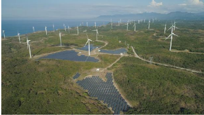
Aerial view of solar farm and windmills for electric power production in Ilocos Norte.
