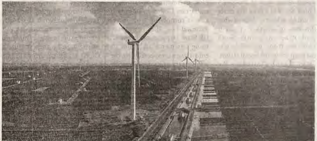
■ Solar power stations in plain areas, wind turbines in the distance. UN PHOTO
