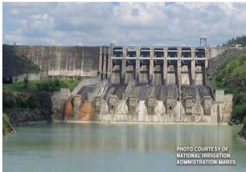
Magat Dam spillway (Photo courtesy of NIA-MARIIS)
