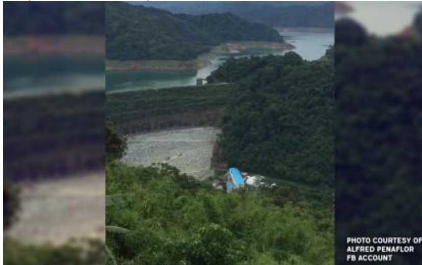
Angat Dam (File photo)
