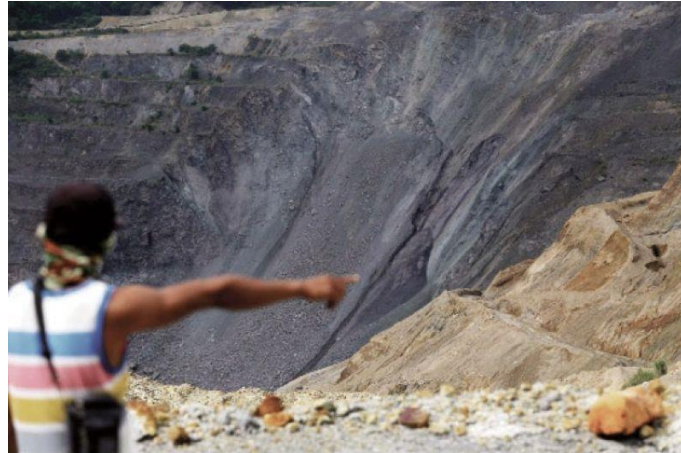
LANDSLIDE SITE. A habal-habal driver points to the crown of the landslide at Carmen Pit in the Toledo copper mines. (Alan Tangcawan)
