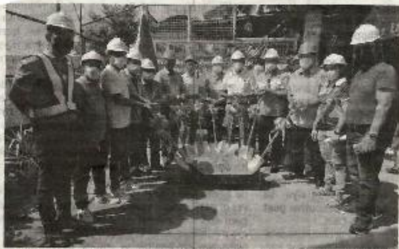
SANITATION INFRA FOR PANAQUE ESTERO. West Zone concessionaire Maynilad Water Services, Inc. (Maynilad), together with the Department of Environment and Natural Resources (DENR), the local government of Parañaque, and the Department of Public Works and Highways (DPWH) recently broke ground to install a sewer interceptor line that will catch wastewater generated by communities along Estero de Tripa de Gallina, thus helping to reduce pollution load to waterways that drain out to Manila Bay. Besides installing this sewer line, Maynilad will also maintain, through regular desludging, the communal septic tank that the DENR and Parañaque LGU will construct for the use of more than 1,000 people living along the estero.
