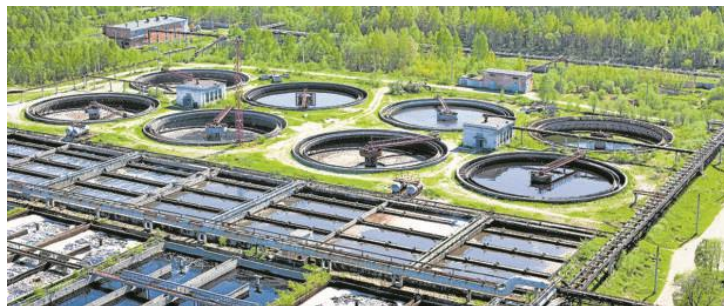
Waste-to-energy facilities used alone or in tandem to operate independently or to complement an existing wastewater treatment system
