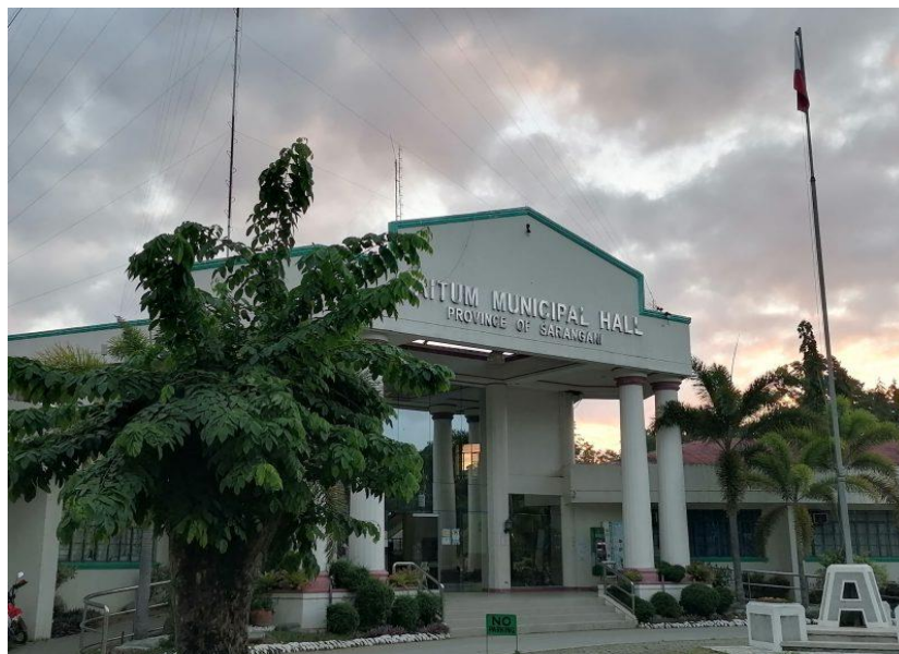
The municipal hall of Maitum, Sarangani on 24 February 2021. MindaNews photo by BONG S. SARMIENTO
