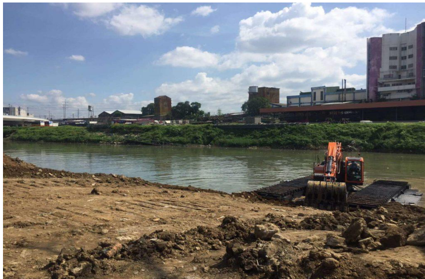
(Photo via DPWH)
