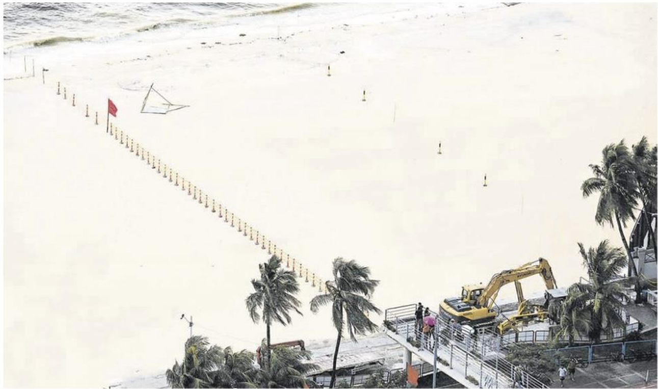
AN AERIAL view of the portion of Manila Bay recently rehabilitated and beautified with crushed dolomite.
