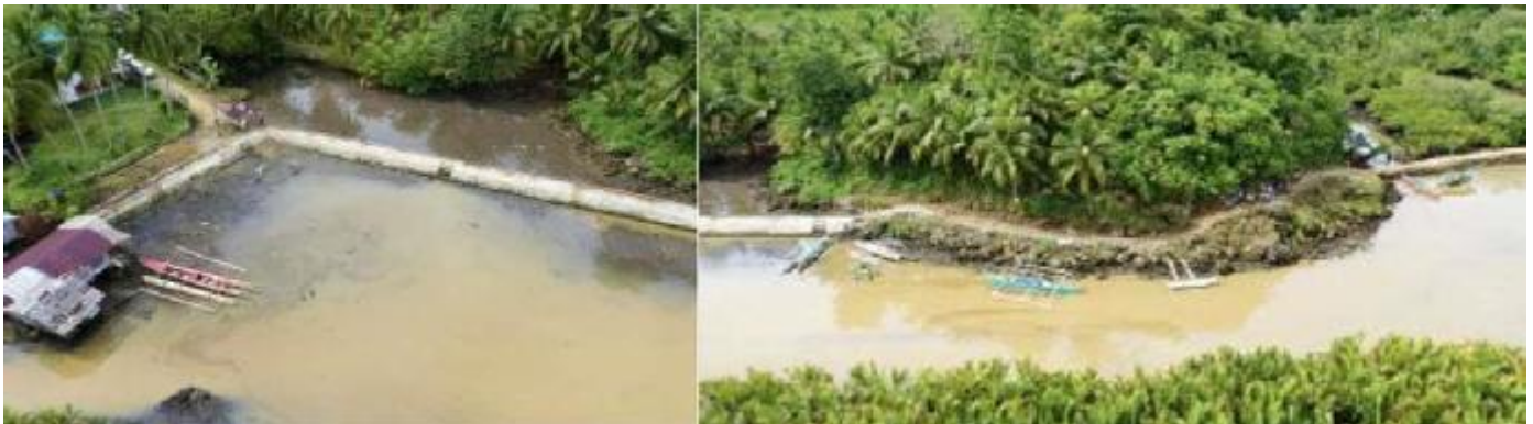
The wharf (right photo) and pathway (left photo) which were constructed under the Department of Social Welfare and Development's (DSWD) KALAHÍ-CIDSS and Risk Resiliency Program (RRP) now serve as barriers to minimize coastal erosion in Barangay San Roque, Pilar, Surigao del Norte.
