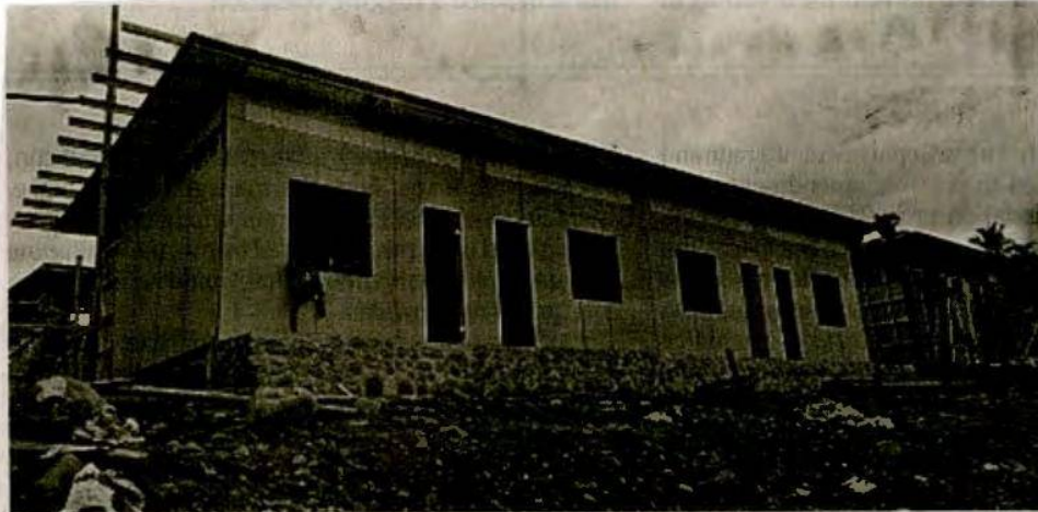
TRANSITION SHELTERS (Photo courtesy of Baybay City Engineering Office)
