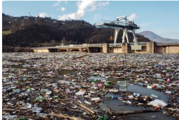
Plastic trash is seen near a dam's hydroelectric plant littering the polluted Potpecko Lake, Serbia, January 5, 2021. Picture taken on January 5, 2021. Branko Filipovic, Reuters
