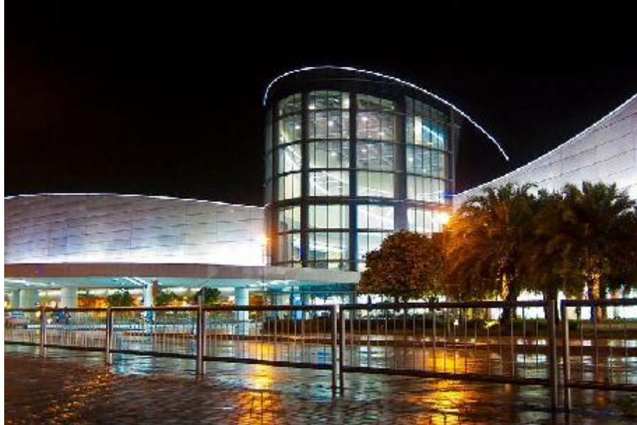
SM Mall of Asia main facade
