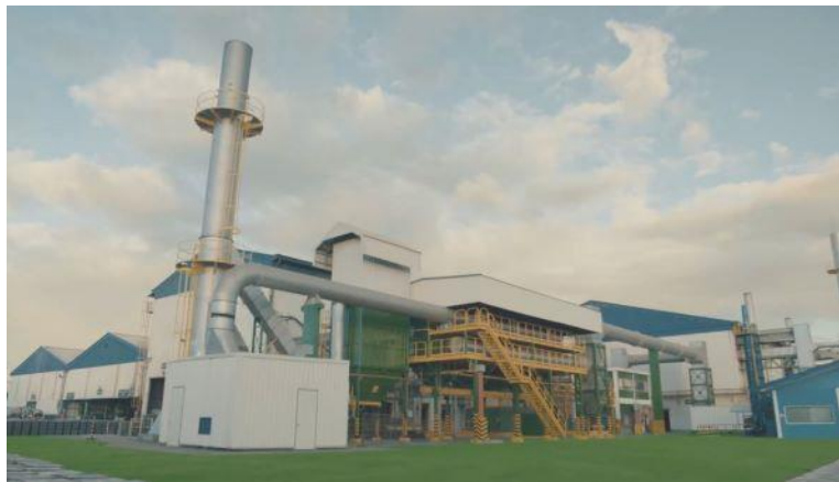
EERI's world-class battery recycling plant
