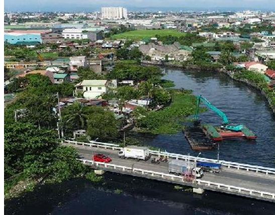
Tullahan River being cleaned up
