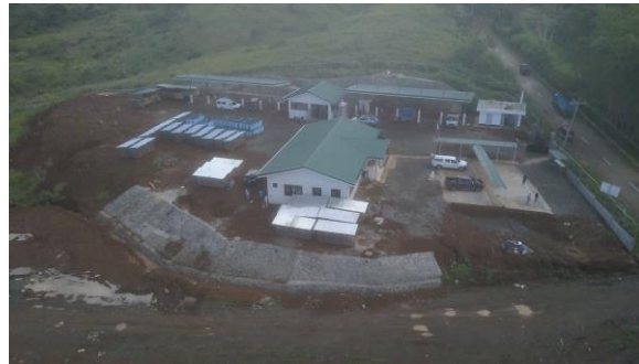
Aerial photo of the administration building, overhauling area, warehouse and storage, and powerhouse with supply, delivery, and installation of 100-KVA standby power/generator set constructed in the 2.2 hectares land for the Task Force Bangon Marawi Solid Waste Management Project. (Angelo Dologmandin/PIA ICIC)
