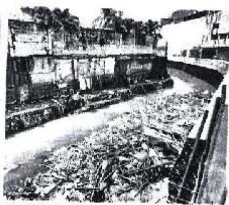
DEBRIS A pile of debris is left along the Kinalumasan River in Cebu City after the demolition of structures in the area on Aug. 8. —PHOTO COURTESY OF THE CEBU CITY PUBLIC INFORMATION OFFICE
