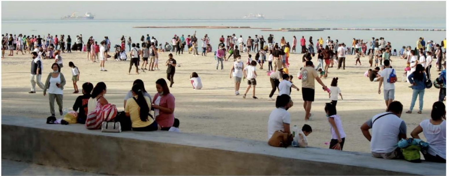
THE still-being-constructed dolomite beach on Manila Bay is an instant hit among city dwellers who have been ensconced in their homes due to the pandemic.
