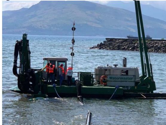
(Photo via DPWH)
