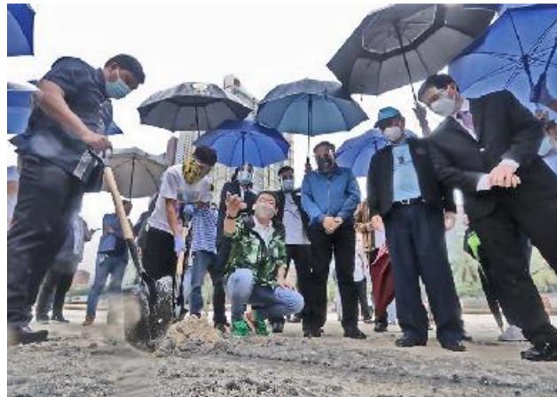
Environment Secretary Roy Cimatu and Supreme Court Chief Justice Diosdado Peralta inspect the Manila Bay white-sand project and the solar-powered sewage treatment plant in Manila on Wednesday. The Chief Justice hailed the progress of the cleanup in compliance with the SC's continuing mandamus.
