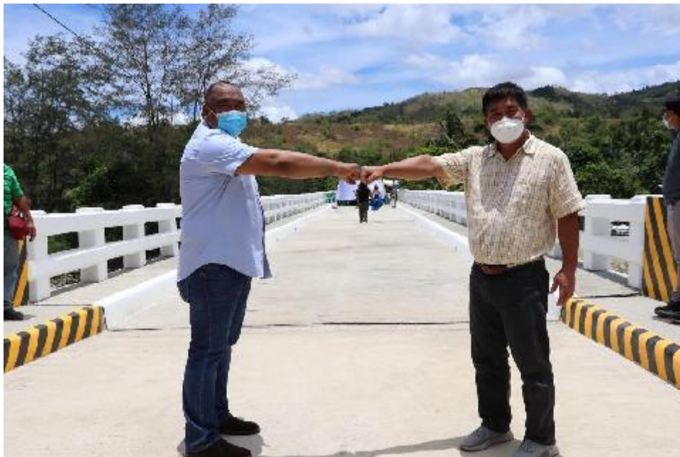
Department of Environment and Natural Resources Regional Executive Director Paquito Moreno Jr. (right) and Pantabangan Mayor Roberto Agdipa (left) lead the inauguration of the 60-meter reinforced concrete deck girder bridge in sitio Pamalayan in barangay Conversion that will be essential to the rehabilitation of the 44,000-hectare Pantabangan-Caranglan Watershed. (DENR)
