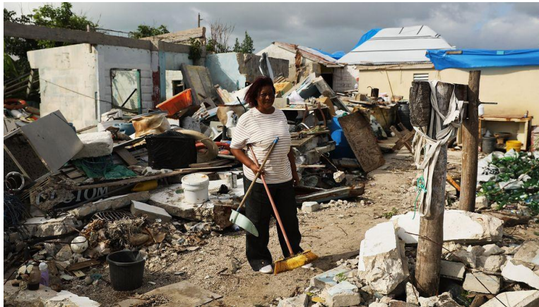
Every single building on Barbuda was damaged by Hurricane Irma, many of them left entirely uninhabitable (Credit: Getty Images)
