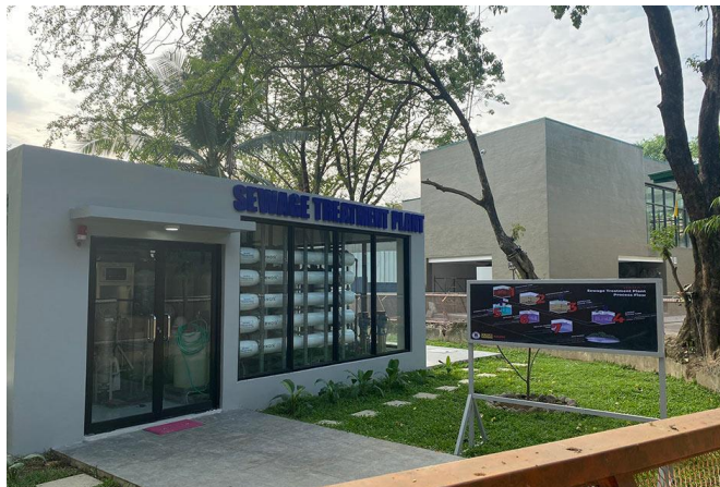
The zoo now has its own Sewage Treatment Plant. Photo: ABS-CBN News
